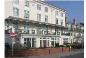
One of the 700 Abbeyfield Houses in The UK Abbeyfield Court Sidmouth, Devon (pict. www.abbeyfield.com )
